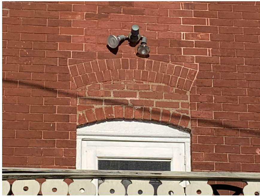
7. EXISTING BRICK DETAIL OVER 1ST FLOOR DECK DOOR
