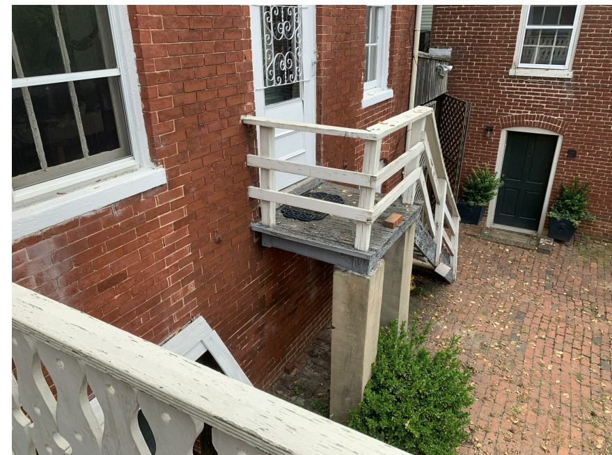
4. COURTYARD ON SOUTH FROM 1ST FLOOR DECK
