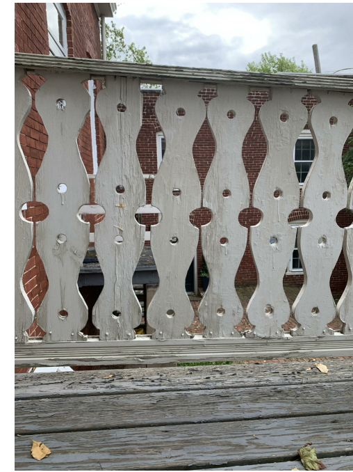
3. DECORATIVE RAILING ON DECK
