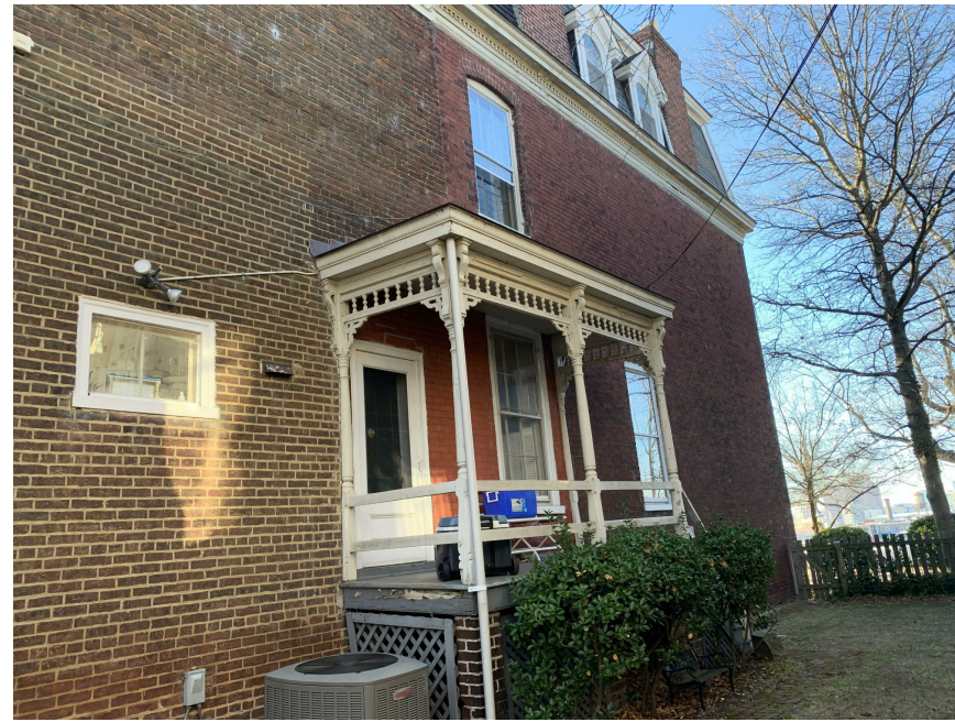
8. VIEW OF PORCH FROM NORTHERN YARD
