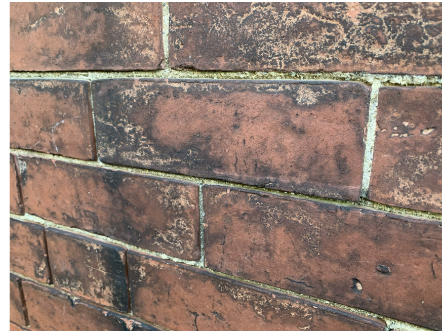
9. EXISTING BRICK DETAIL ON NORTH SIDE
