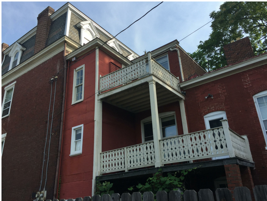
1. SOUTHEAST VIEW OF DECKS
