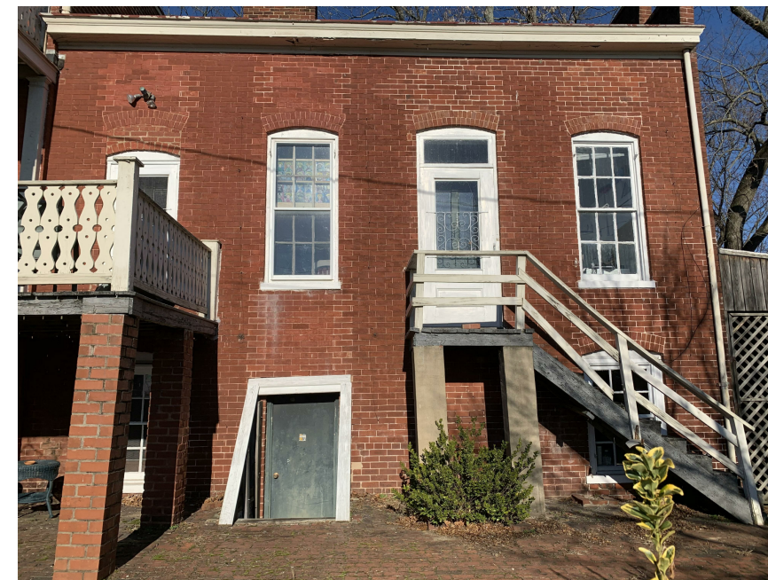
6. VIEW FROM SOUTH COURTYARD
