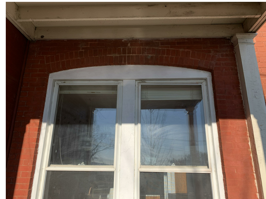
12. EXISTING 1ST FLOOR DECK WINDOWS
