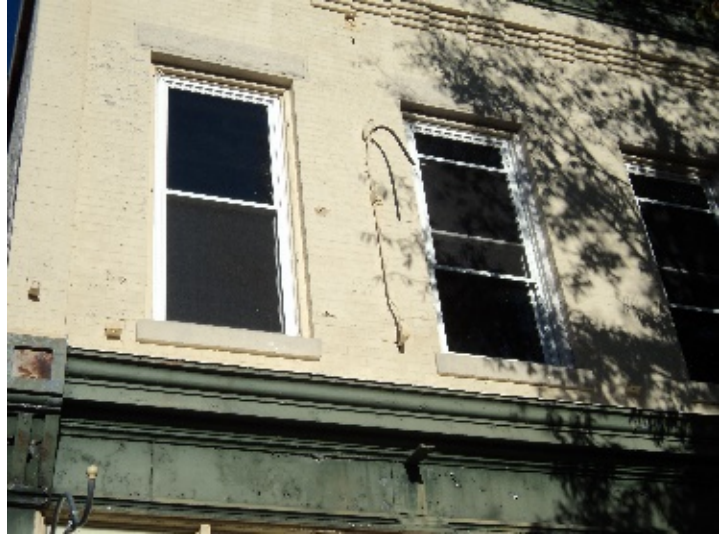
Figure 6. Replacement windows, facade.
