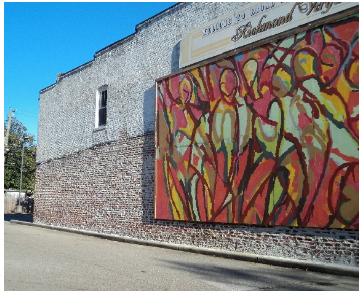
Figure 4. Side wall, 508 W. Broad Street
