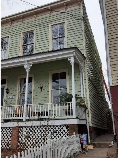
Figure 1. Front façade of 413 N. 27 th Street
