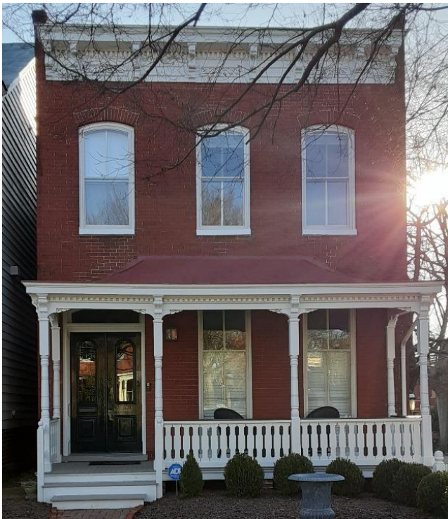
Figure 1. Front façade of 2701 E. Grace St.
