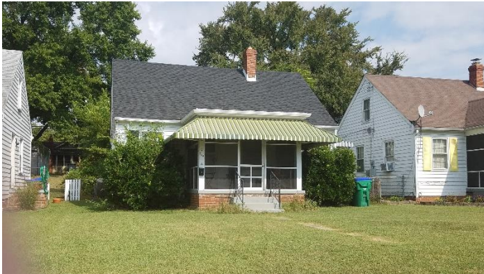
Figure 1. 509 West 22nd Street, façade
