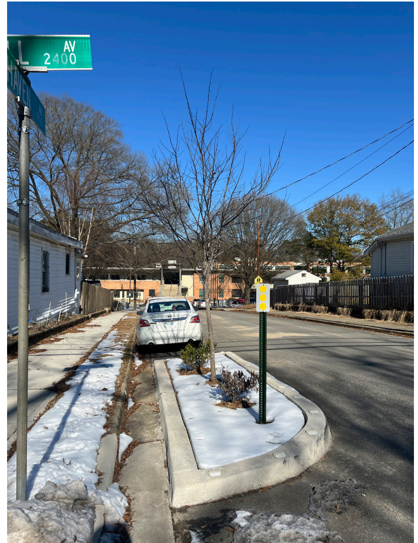
Intersection improvements at Lynhaven and Royall Avenues. The curb bumpouts slow drivers and add a small space for vegetation.
