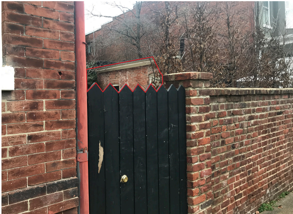
4 - VIEW OF WEST FACADE OUTLINED IN RED (WINTER)
