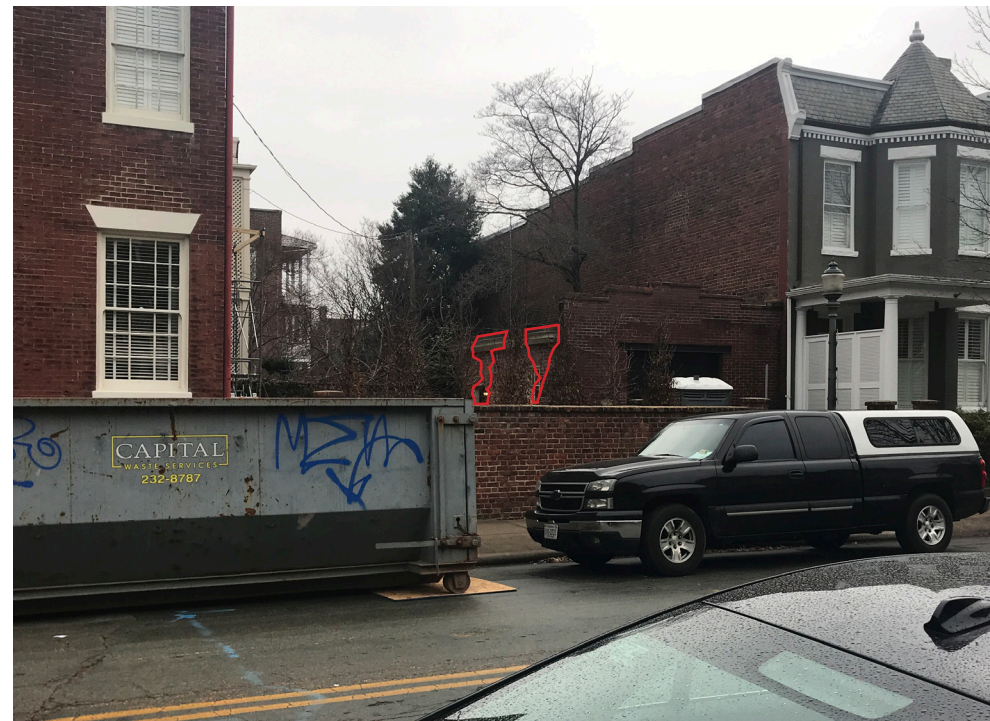
5 - VIEW OF WEST FACADE OUTLINED IN RED (WINTER)
