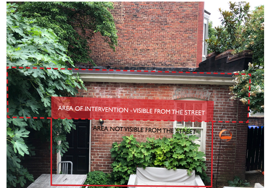
6 - AREA OF INTERVENTION WHICH IS VISIBLE FROM THE STREET
