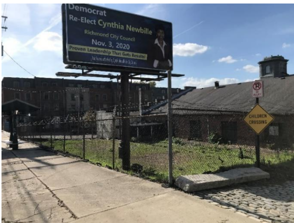
Figure 5. 304 North 21st Street from 21st Street
