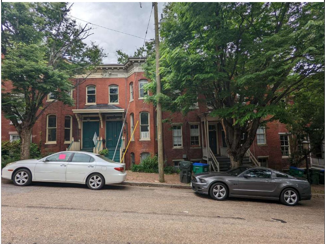
NEIGHBOR (LEFT) OF PROJECT HOUSES
