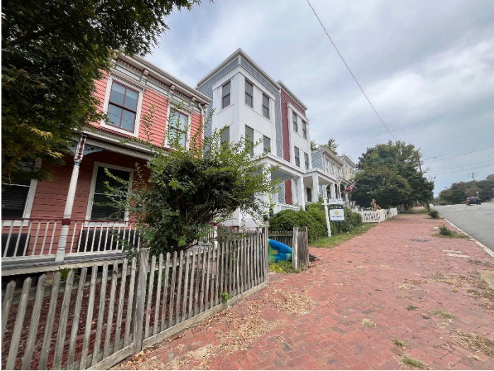
Figure 3. Context, Looking east down E. Broad St.
