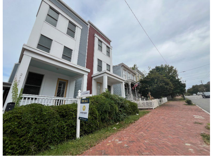
Figure 4. Other new construction on subject block.
