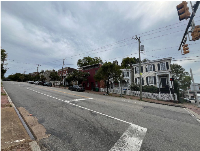
Figure 5. Context. South side of 2100 Block E. Broad.
