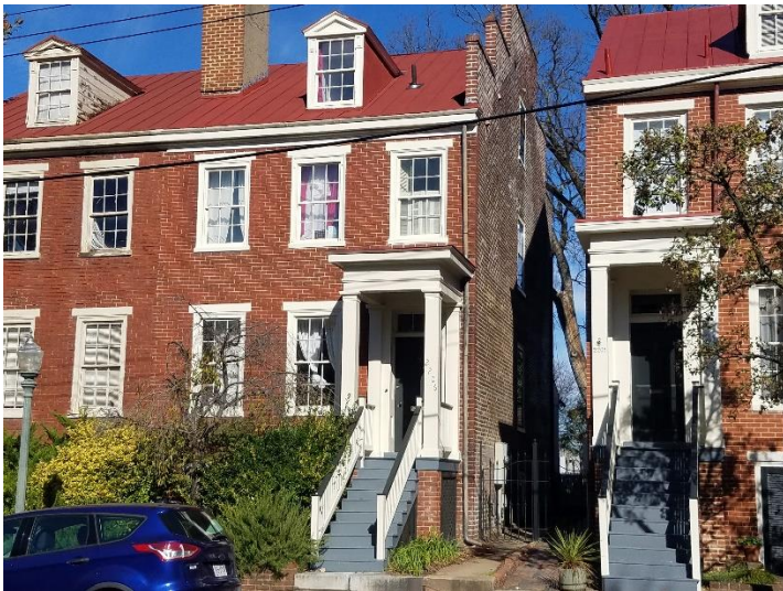
Figure 3. 2206 East Broad Street.
