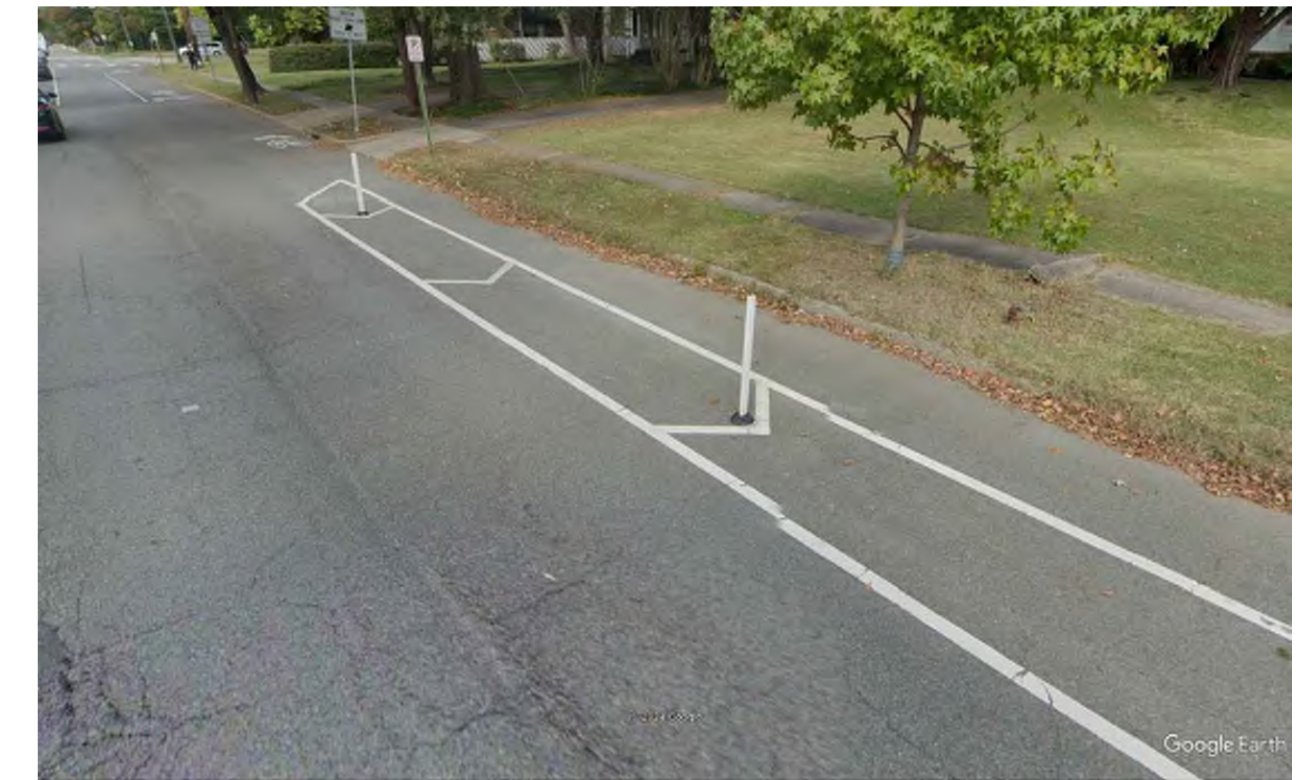
TYPICAL PAVEMENT MARKING & FLEXIBLE POST / BOLLARD INSTALLATION IMAGE FROM: BROOK ROAD, CITY OF RICHMOND
