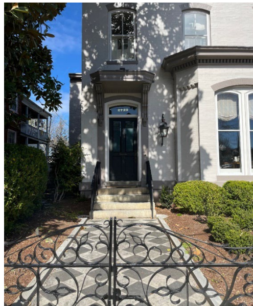
Figure 2. 2720 East Broad Street. Primary Entrance. Location of new balustrade.
