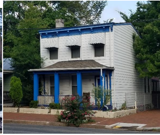
Figure 8. 422 North 26th Street.
