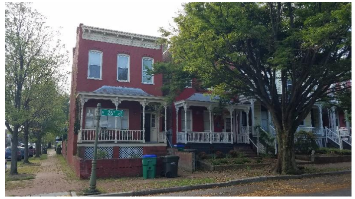
Figure 10. 425 and 427 North 26th Street.
