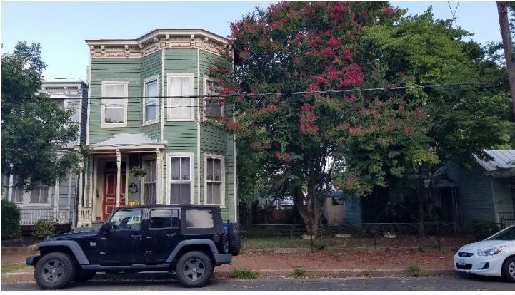
Figure 7. 418 and 416 North 26th Street.
