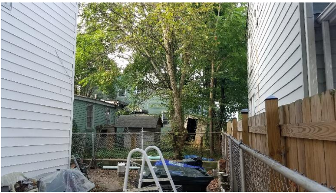
Figure 3. 420 North 26th Street, rear elevation. View from East Clay Street.
