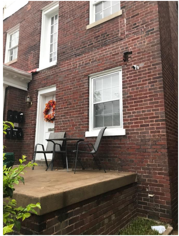
Figure 6. Evidence of ghost lines and previous column locations.
