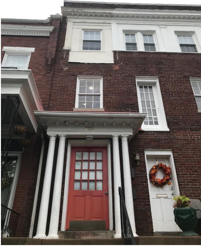
Figure 5. Existing columns surrounding the entryway.
