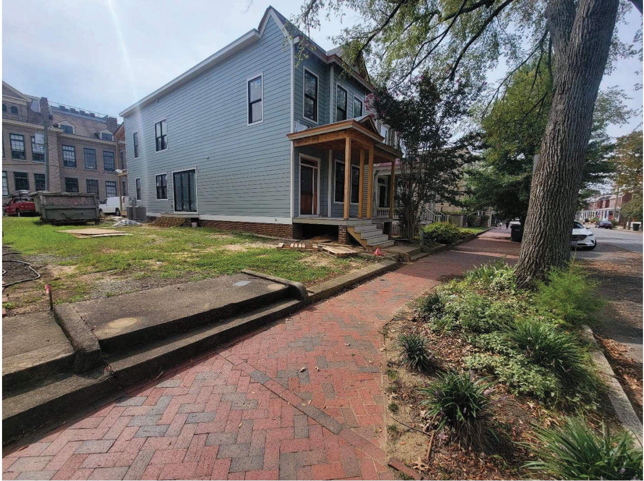
Existing concrete wall and steps to a house that demolished years ago
