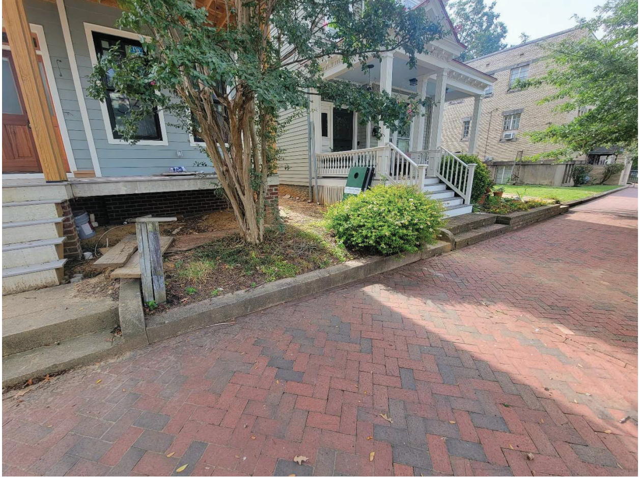
Existing concrete wall in front of 313 N. 32 nd St. and existing brick wall and steps/walk in front of 311 N. 32 nd St.
