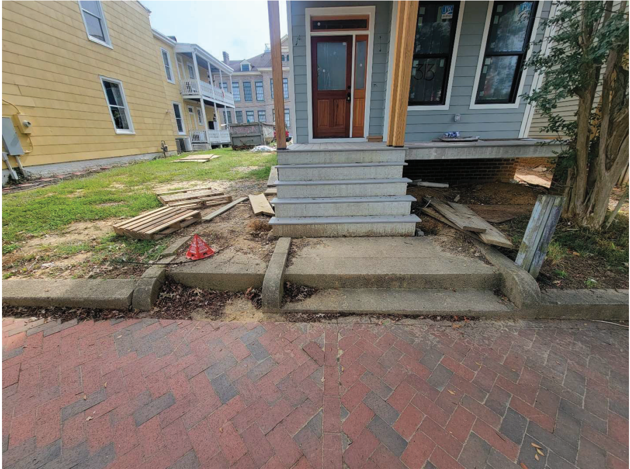
The existing concrete retaining wall as step/walk.
