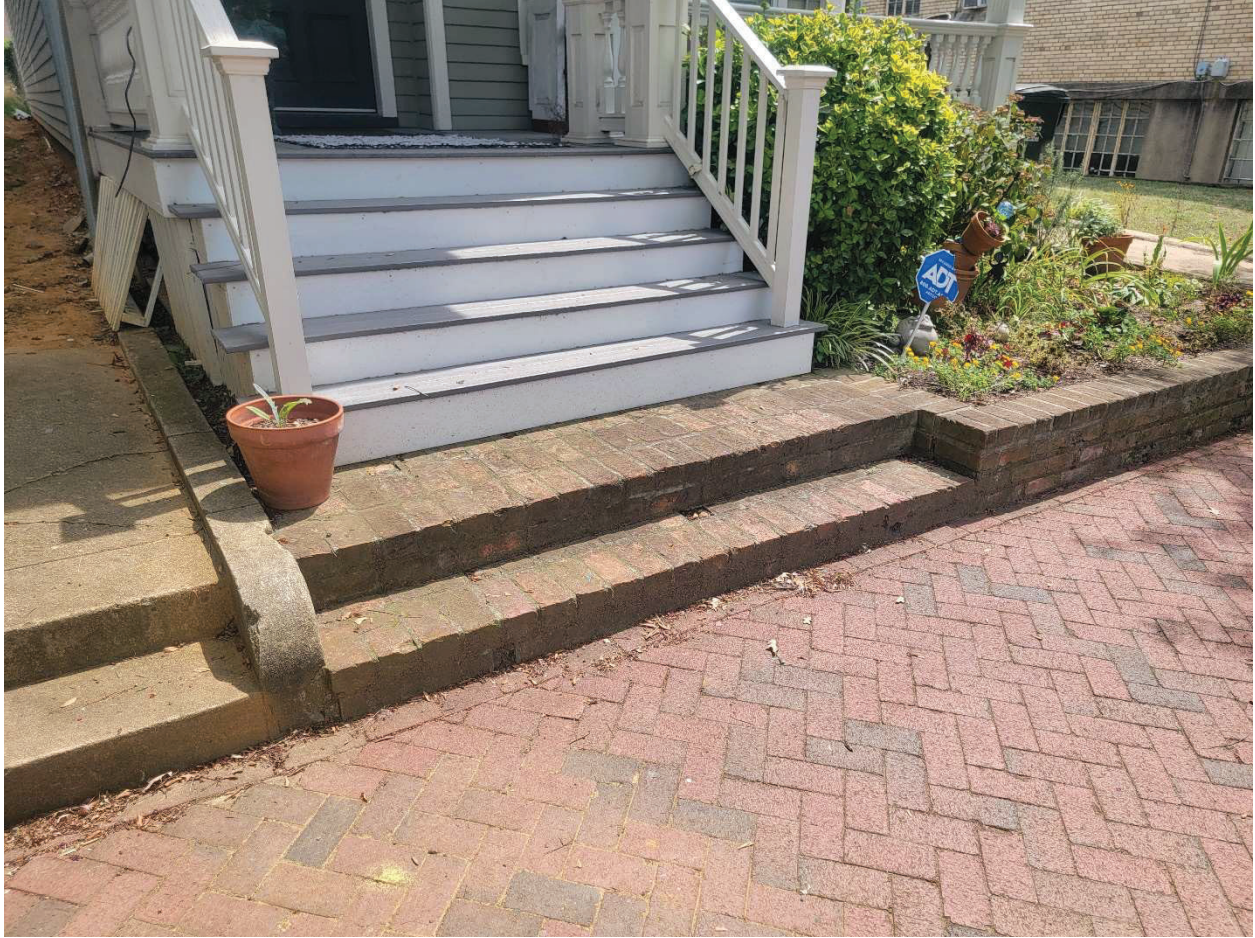
Existing brick wall and steps/walk at 311 N. 32 nd St.
