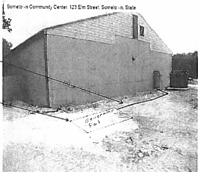
Figure 4. Ground-level photograph showing proposed ground disturbance area.
