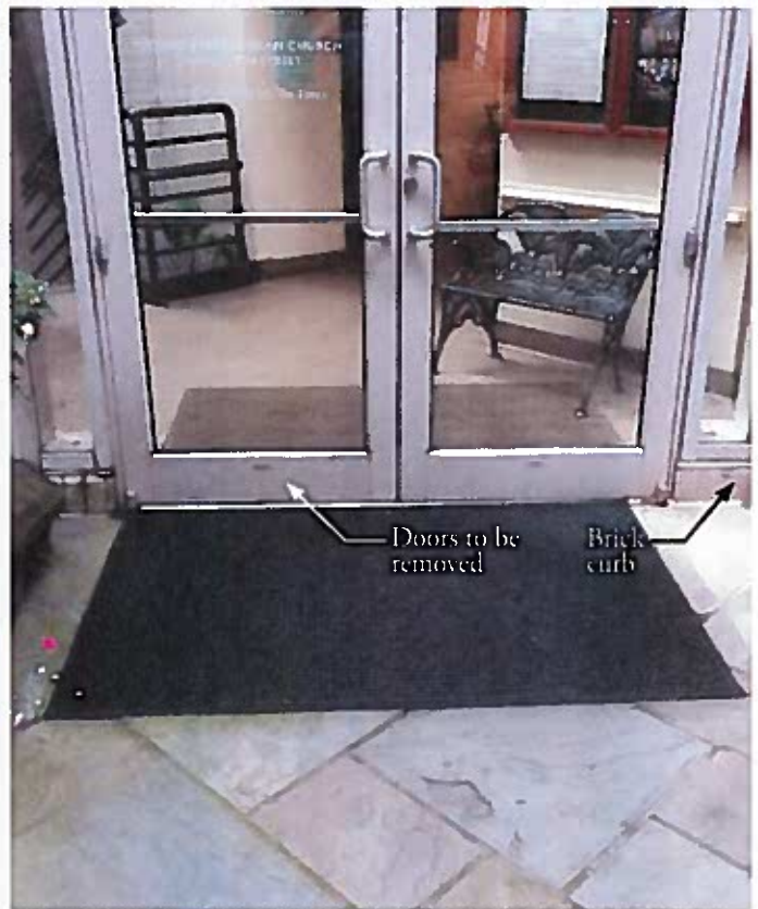
VIEW FROM COURTYARD OF EXISTING DOOR AND PAVERS TO BE REMOVED; BRICK CURB PROFILE TO BE REPLICATED AT NEW CURTAINWALL SILL
