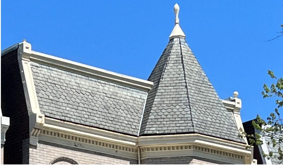
Figure 2. Existing Slate roof. Design
