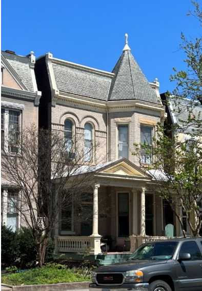
Figure 1. 1634 W. Grace Street Front Facade
