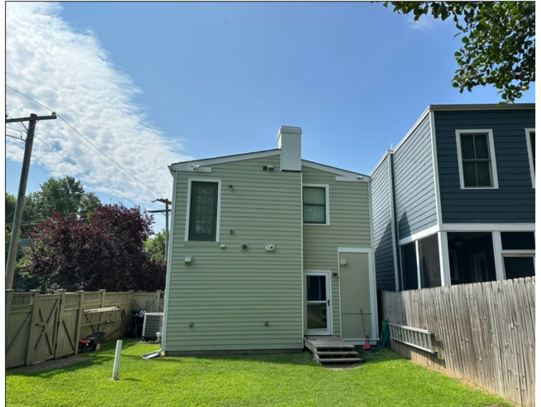
Rear view of main dwelling to illustrate roof slope 2.5/12 (12 degrees). ADU roof slope to match.
