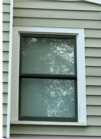
Existing Window on Main Dwelling
