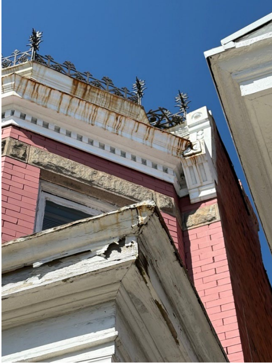
Figure 5. Built-in gutter detail.
