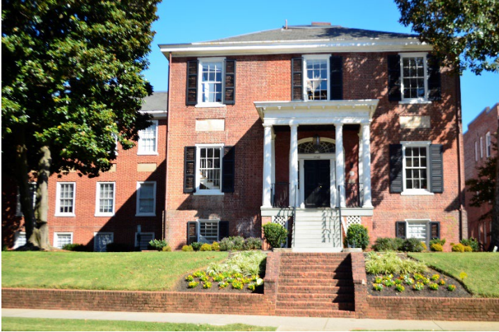
Figure 1. Façade, south side of 1142 West Grace Street
