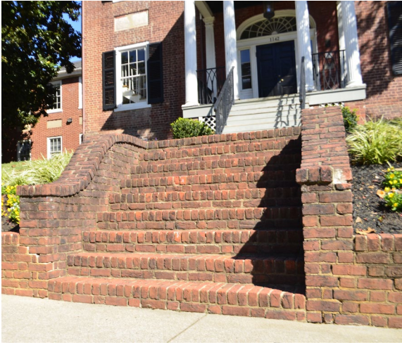
Figure 5. Brick staircase located in front of the West Grace Street entrance of 1142 West Grace Street. The new staircase proposed for this project will be similar to this staircase.
