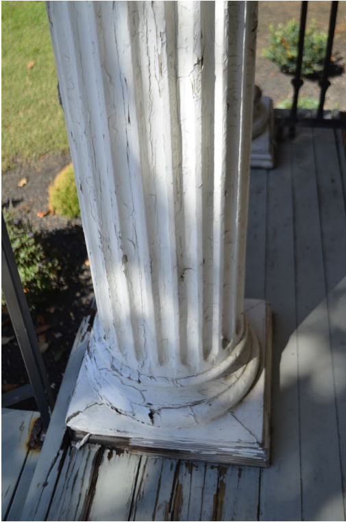
Figure 9. View of deteriorated wooden deck boards and a deterioration at the bottom of the southwest column. The owner plans to repair the deck boards and column with in-kind materials.
