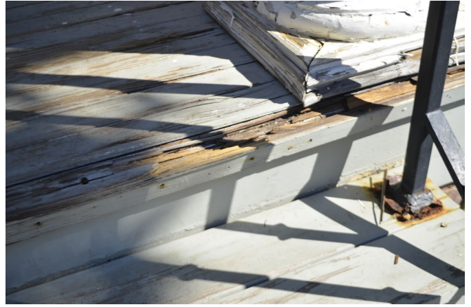
Figure 10. View of the southeast column and further deterioration of the deck boards.
