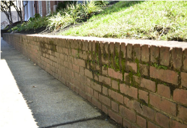
Figure 7. View of the brick wall on the west side of the property. The wall will be repaired and retained after the new staircase is added to the wall.
