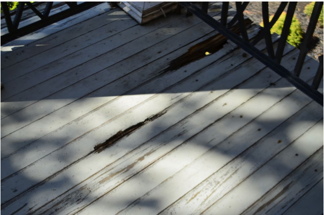
Figure 8. View of deteriorated wooden board on the porch facing Grace Street. This porch will be repaired with in-kind materials.
