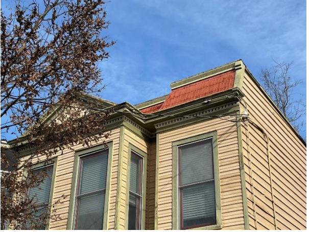
Figure 3. Embossed tin roof at 2208 E. Marshall Street, which is like the original roof of 2206 E. Marshall Street.
