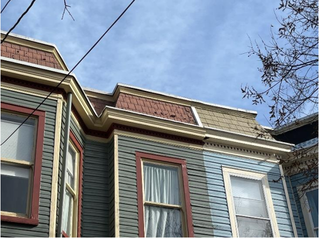
Figure 3. Embossed tin roof at 2208 E. Marshall Street, which is like the original roof of 2206 E. Marshall Street.
