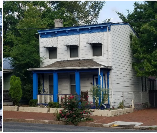
Figure 8. 422 North 26th Street.
