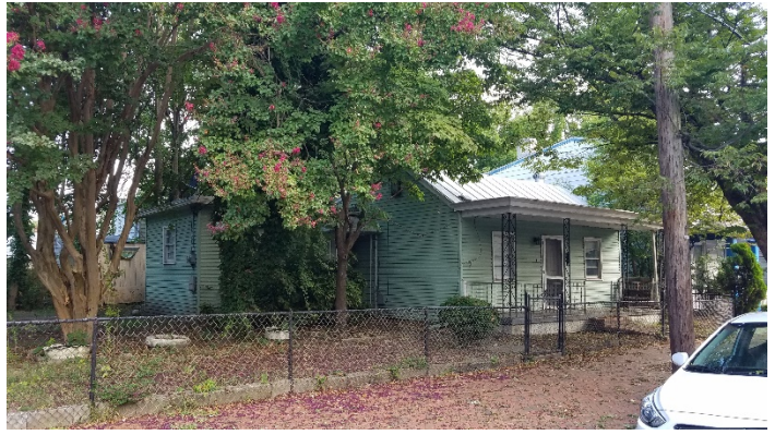
Figure 2. 420 North 26th Street, side addition.
