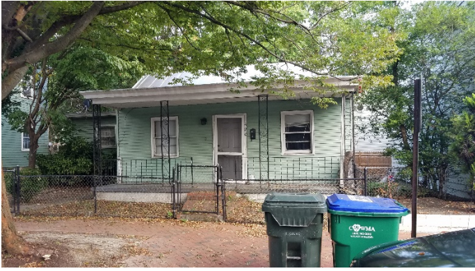
Figure 1. 420 North 26th Street, façade.
