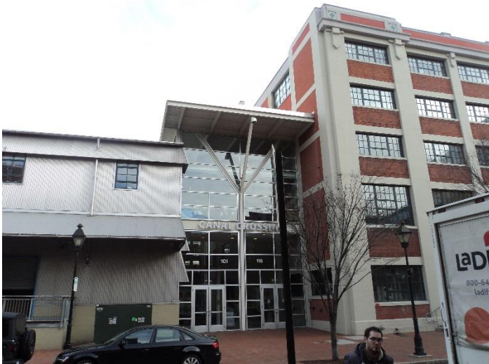
Figure 3. 101 South 15th Street, existing entrance.
