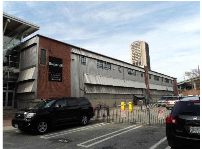
Figure 4. 101 South 15th Street, side elevation.
