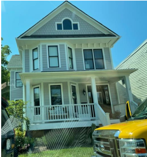
Figure 4 CAR approved new construction 2317 Carrington Street
