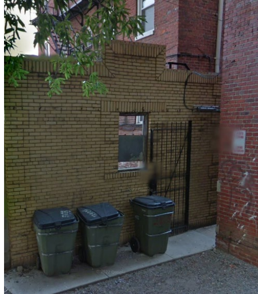
Figure 2. 2011 image of existing wall and window.
