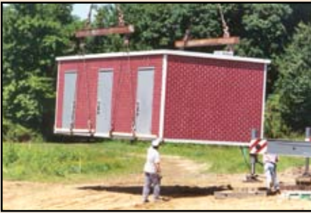
Restroom installation with wet hook ups
