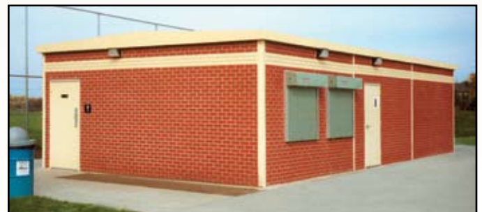
Skyline restroom & concession with Easi-Span roof
