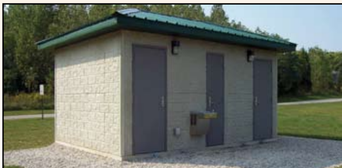
Sierra double restroom with split block finish
