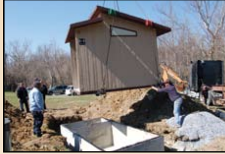
Restroom installation with vault
