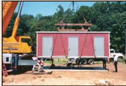
Restroom installation with wet hook ups
