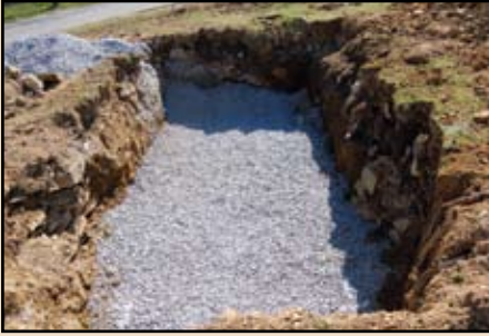
Restroom installation with vault
