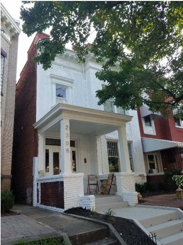
Figure 1. Primed façade of 2306 West Grace Street.
