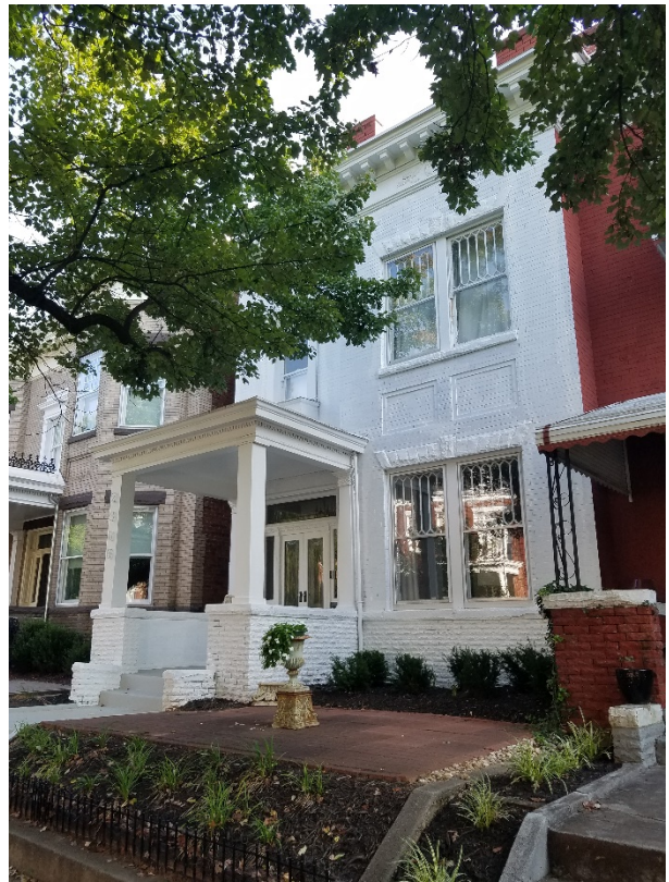
Figure 2. Primed façade of 2306 West Grace Street.
