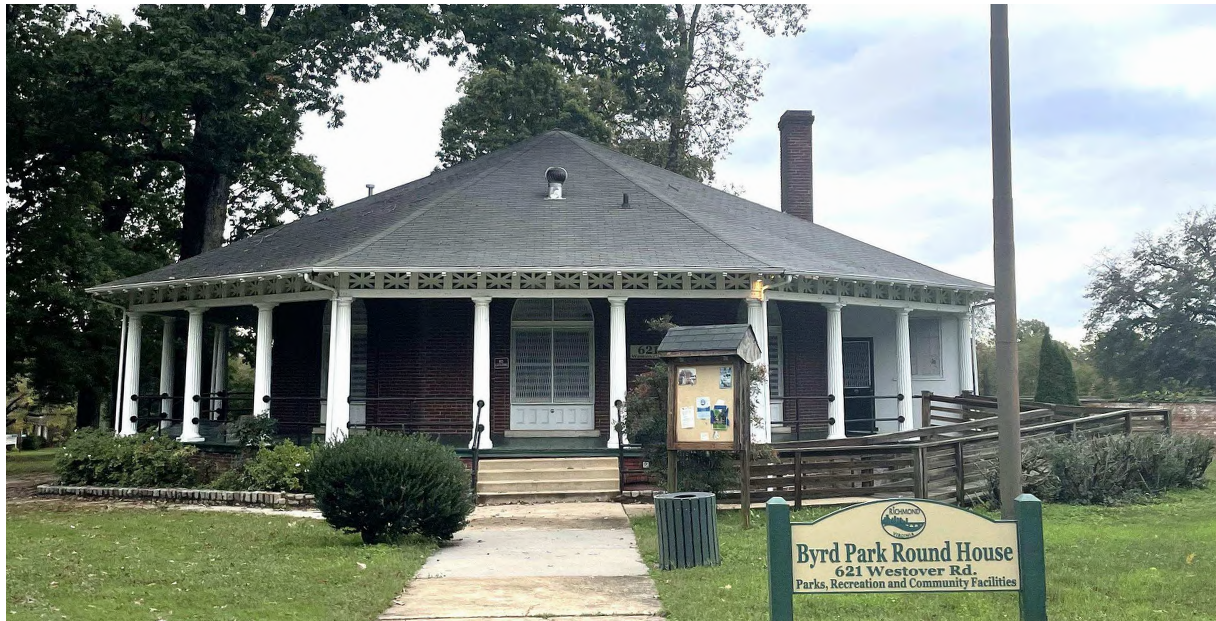
EXISTING WEST FACADE
