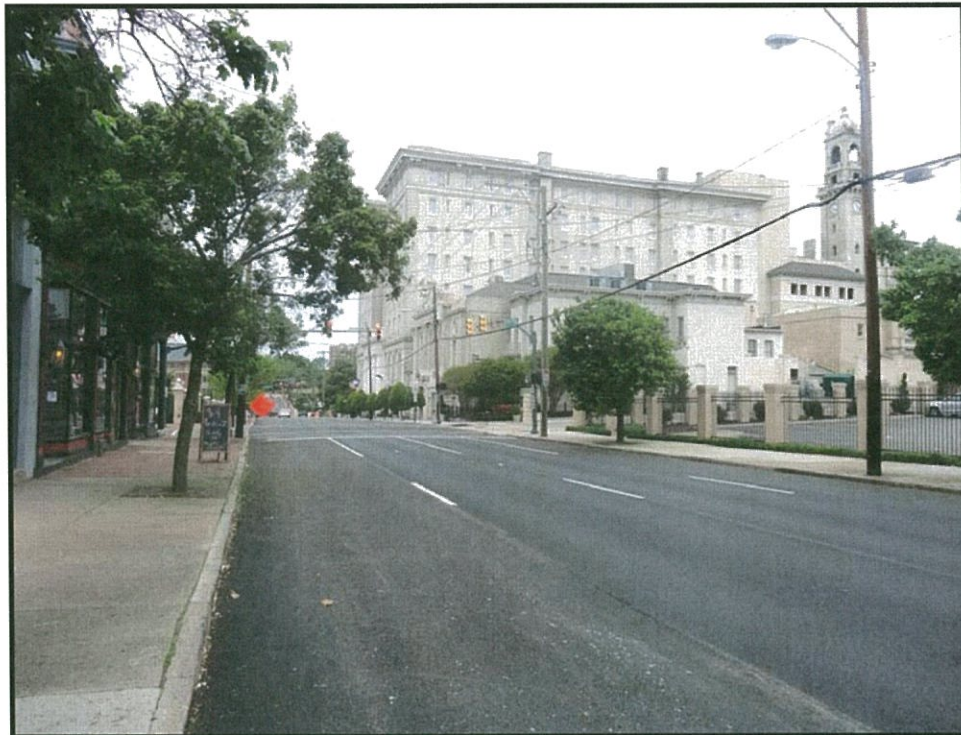
VIEW LOOKING WEST ON MAIN STREET FROM FOUSHEE STREET
