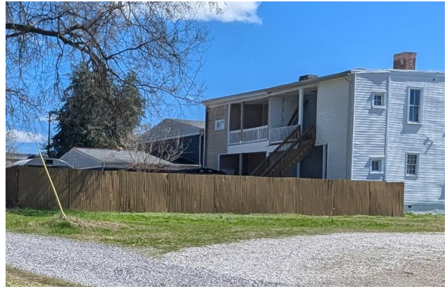
Figure 2. View of rear of 2208 & 2210 Venable Street as seen from North 22 nd Street. March 2026.
