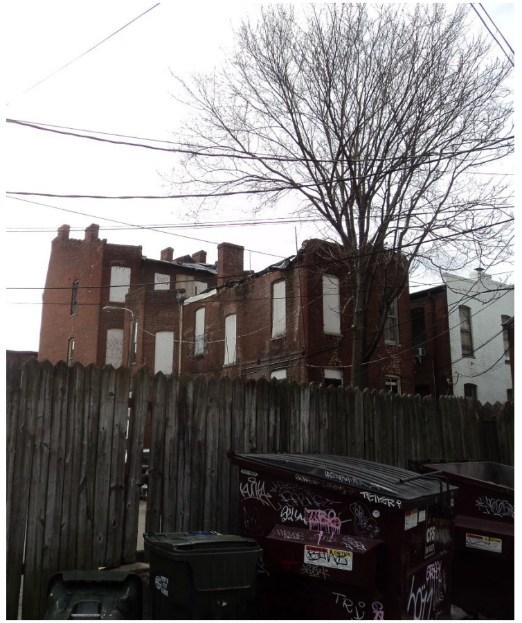
Figure 2. Current view of rear and side elevation
