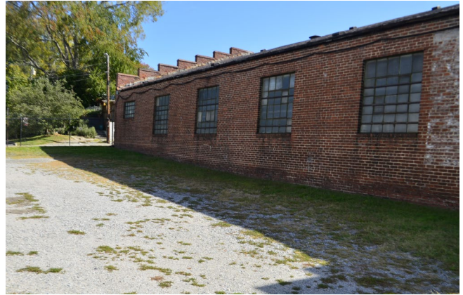
Figure 2. West side of the Repair Shop at 2018 East Broad Street.
