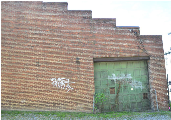
Figure 11. View of the garage door on the north side of the building. This garage door and the one on the south side will be replaced. The applicant plans to add a pedestrian door and a window, east of this garage door.
