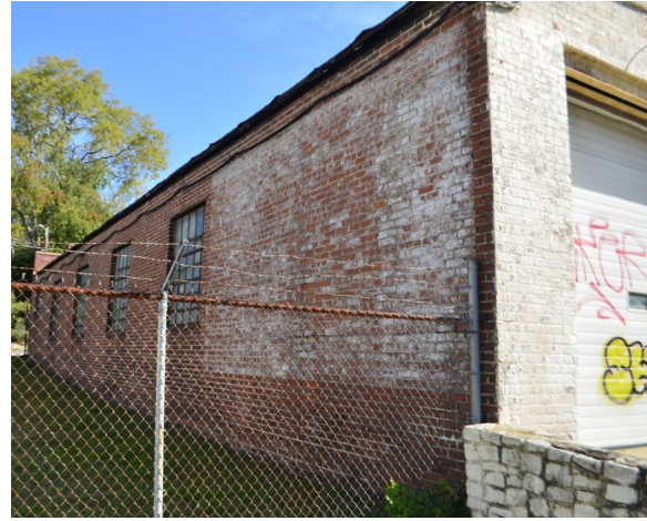
Figure 14. Small masonry wall at the southwest corner of the building. This wall will be replaced with a low, brick wall.
