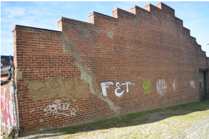
Figure 3. North side of the Repair Shop at 2018 East Broad Street.
