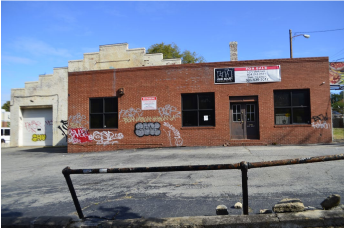
Figure 1. Façade, south side of the Repair Shop at 2018 East Broad Street.
