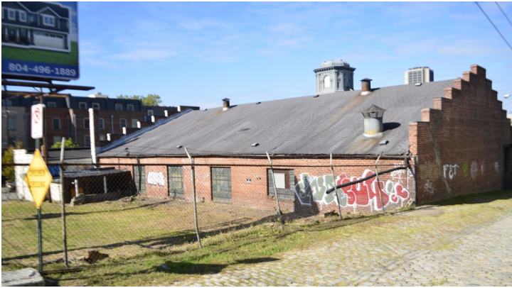
Figure 7. View of the east and north sides of 2018 East Broad Street, from the public alley.
