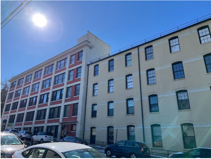
Figure 7. Large -scale historic buildings near the subject site.
