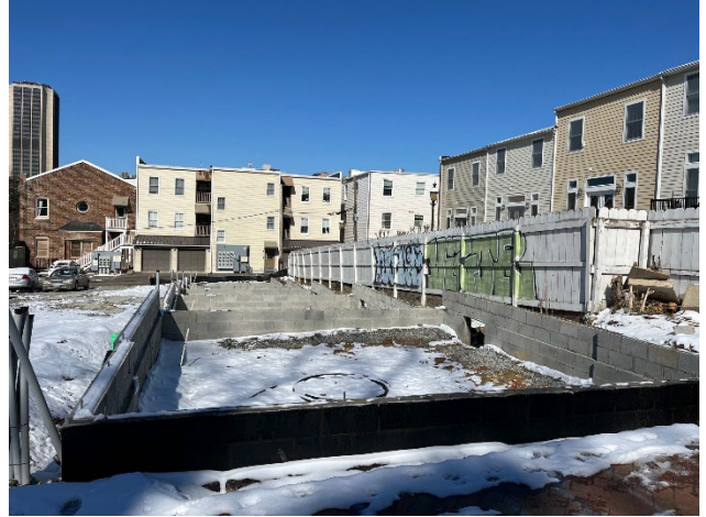
Figure 2. Looking south on east side of North 20 th Street.
