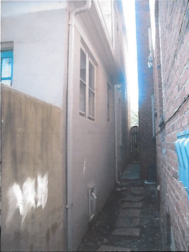
Figure 3: View of north side of property as seen from the rear.
