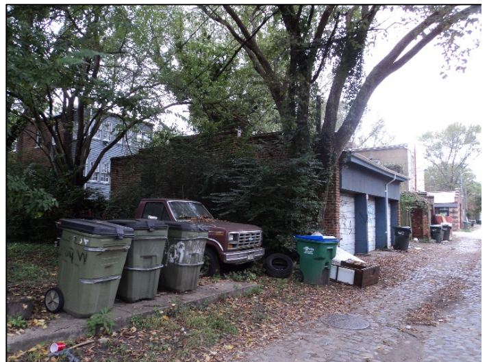
Figure 4. 412 W. Marshall Street, outbuilding facade.
