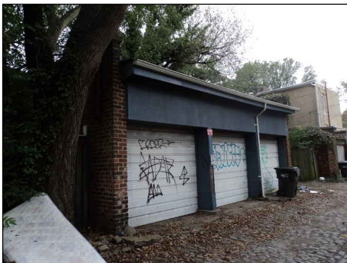
Figure 5. 412 W. Marshall Street, outbuilding facade.
