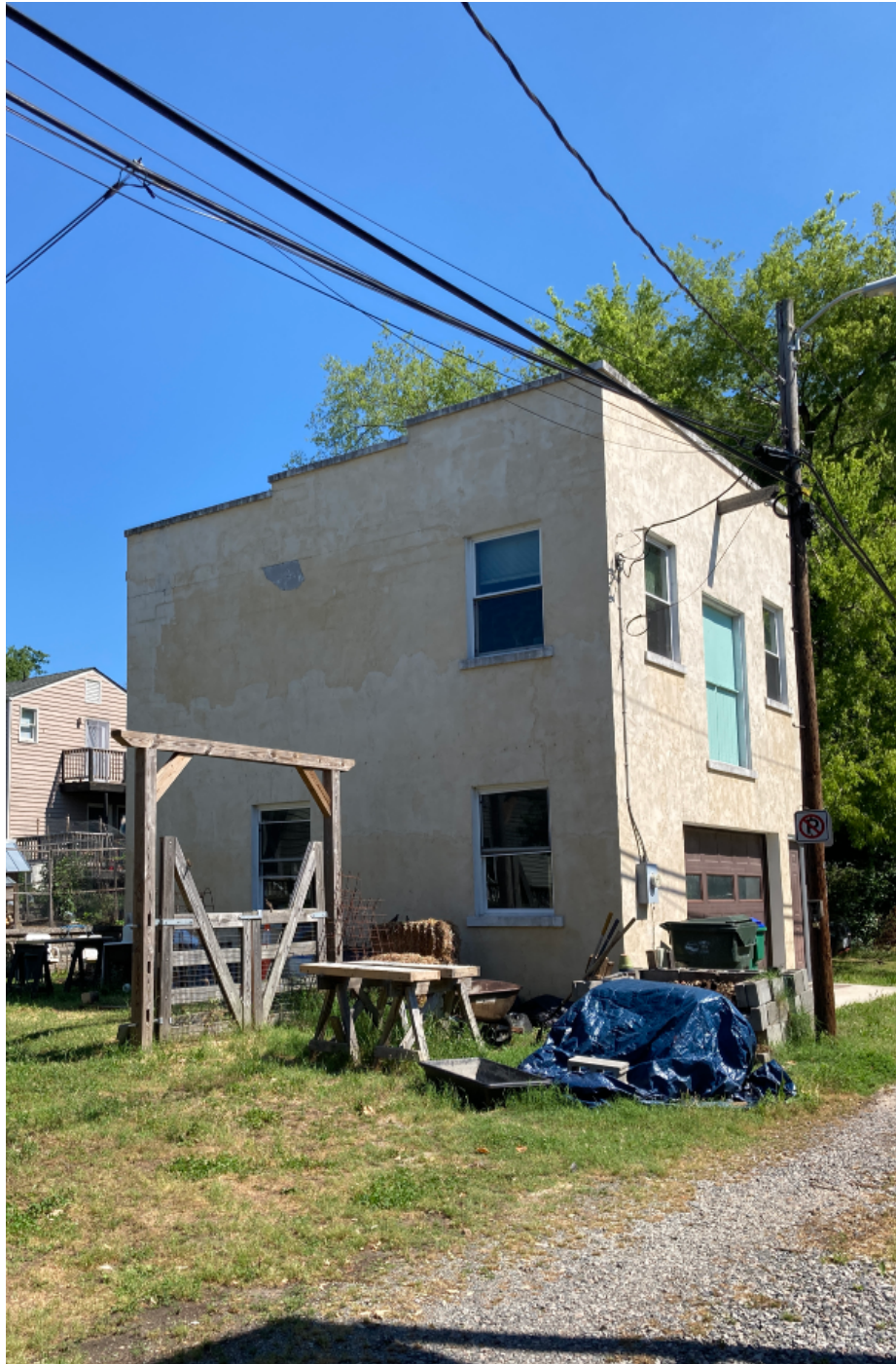
607 N 23rd St. - View from Alley
