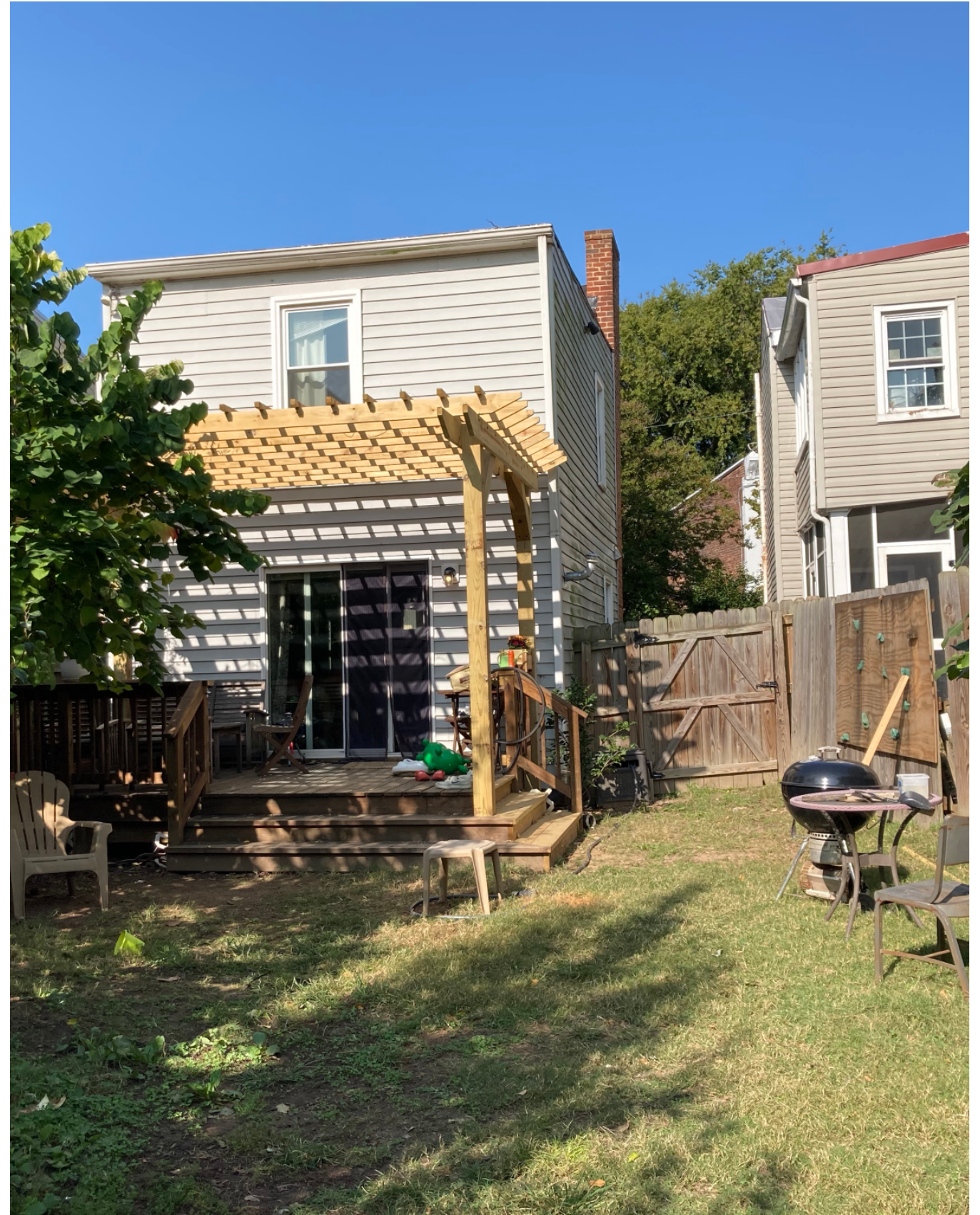
605 N 21st St. - East Elevation
