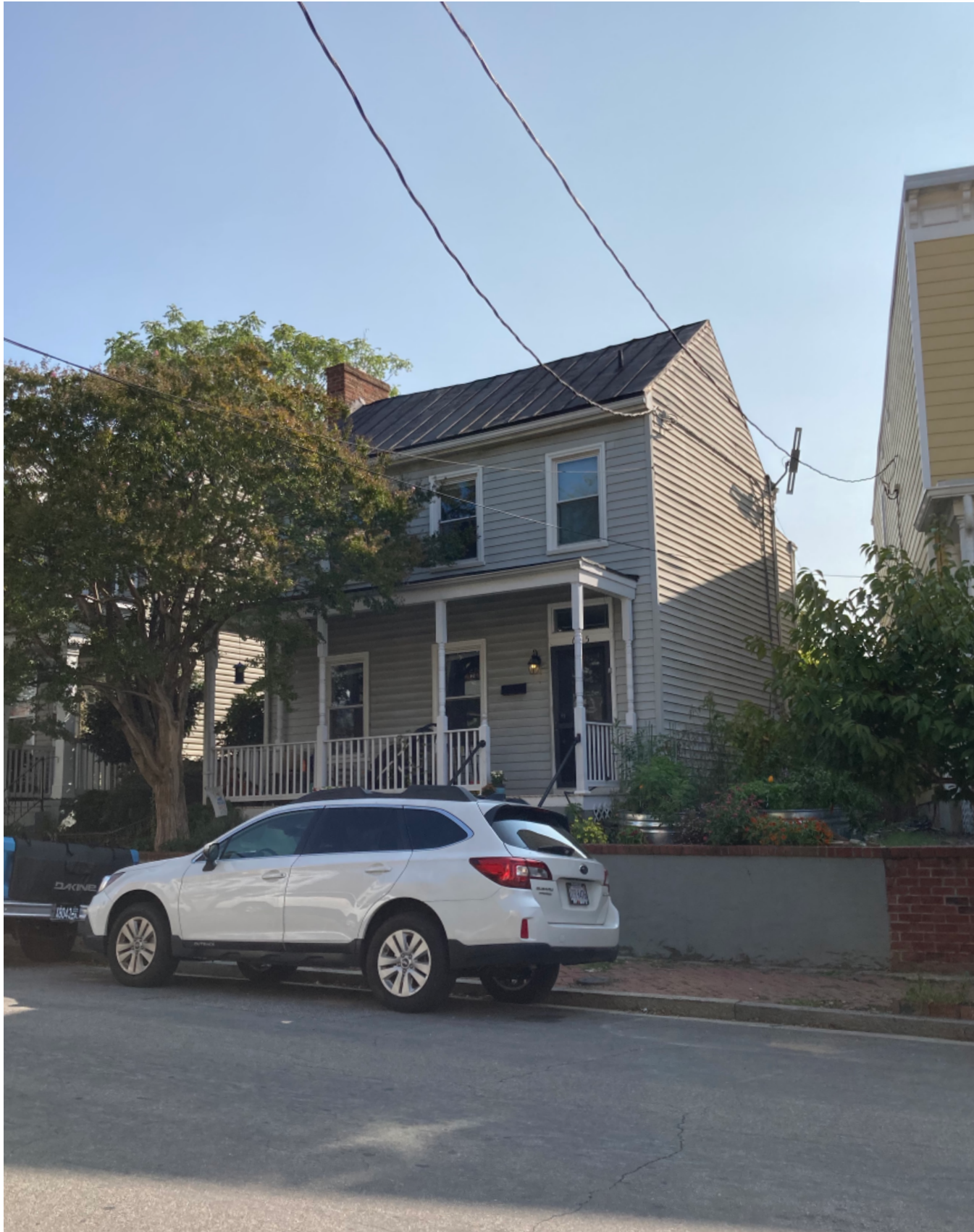
605 N 21st St. - West Elevation
