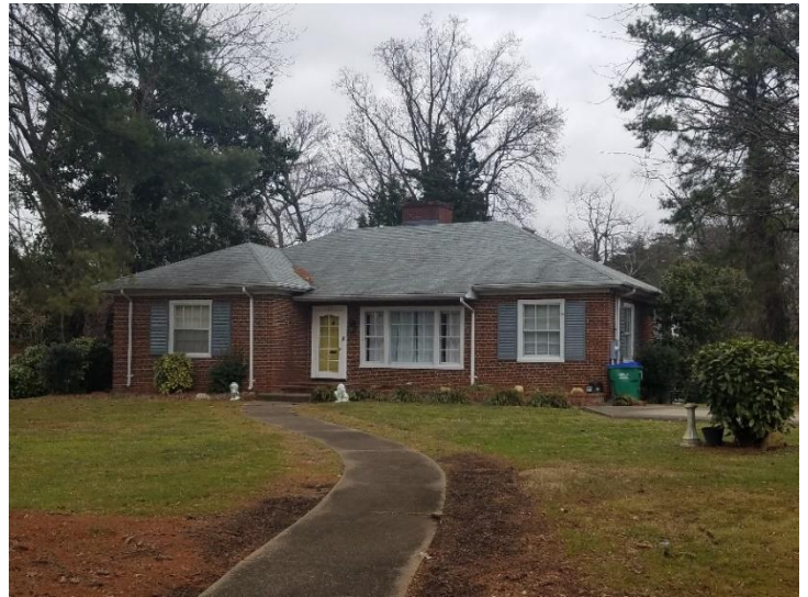
Figure 2. 4201 Hermitage Road, façade
