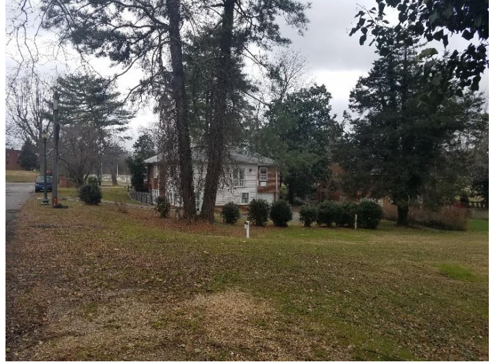
Figure 4. Rear elevation, as viewed from Princeton Road
