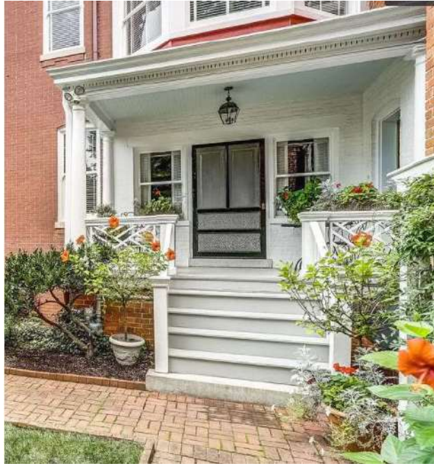
Figure 4. Existing photo of the rear porch proposed to be enclosed.
