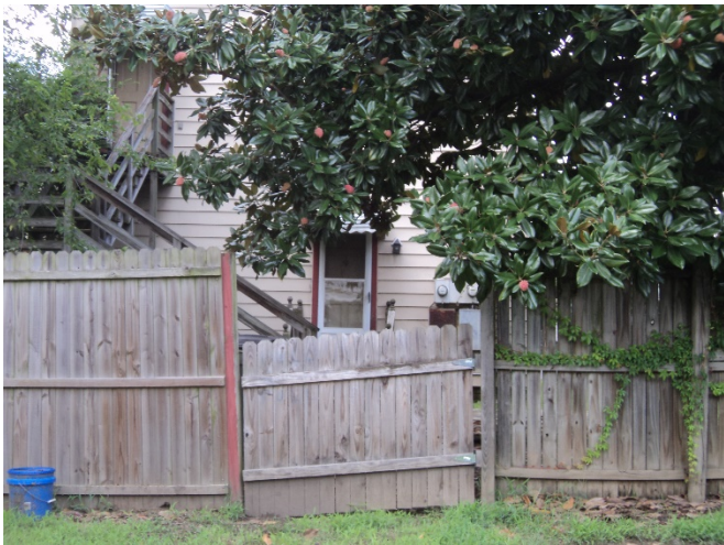
Figure 5. Existing first-story door opening.
