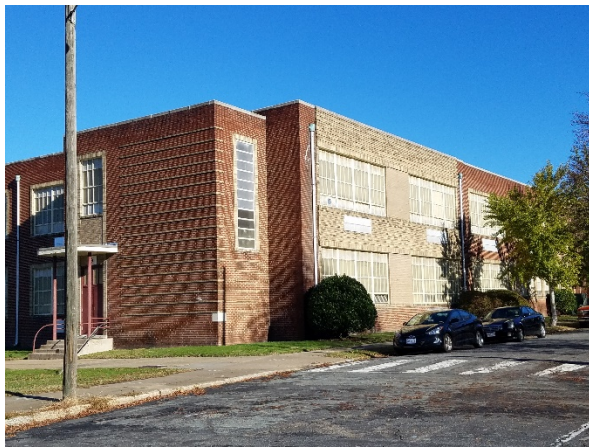
Figure 5. Existing Building, Addition.
