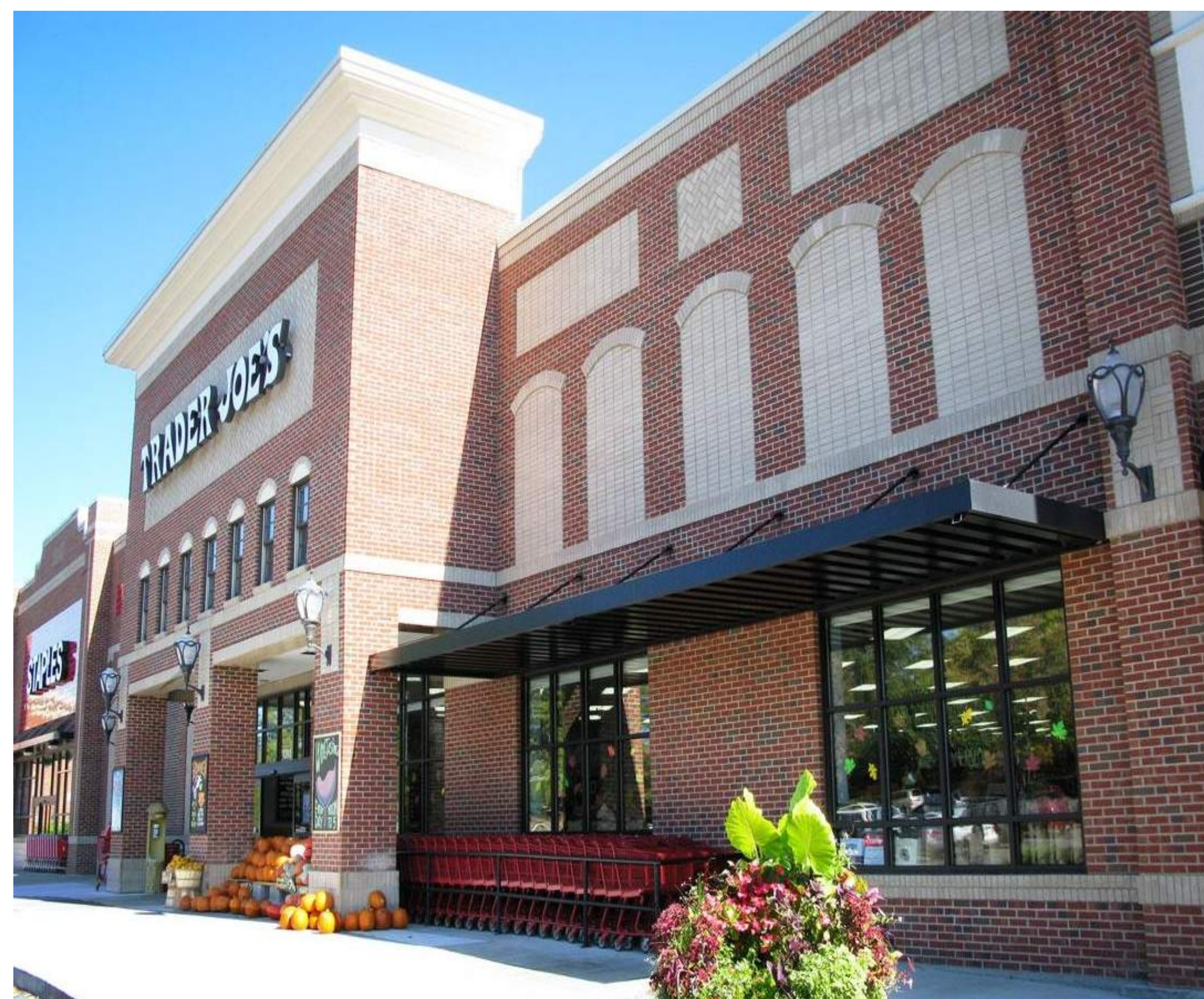
EXAMPLE: - BRICK - PREFINISHED ALUMINUM CANOPY SYSTEM
