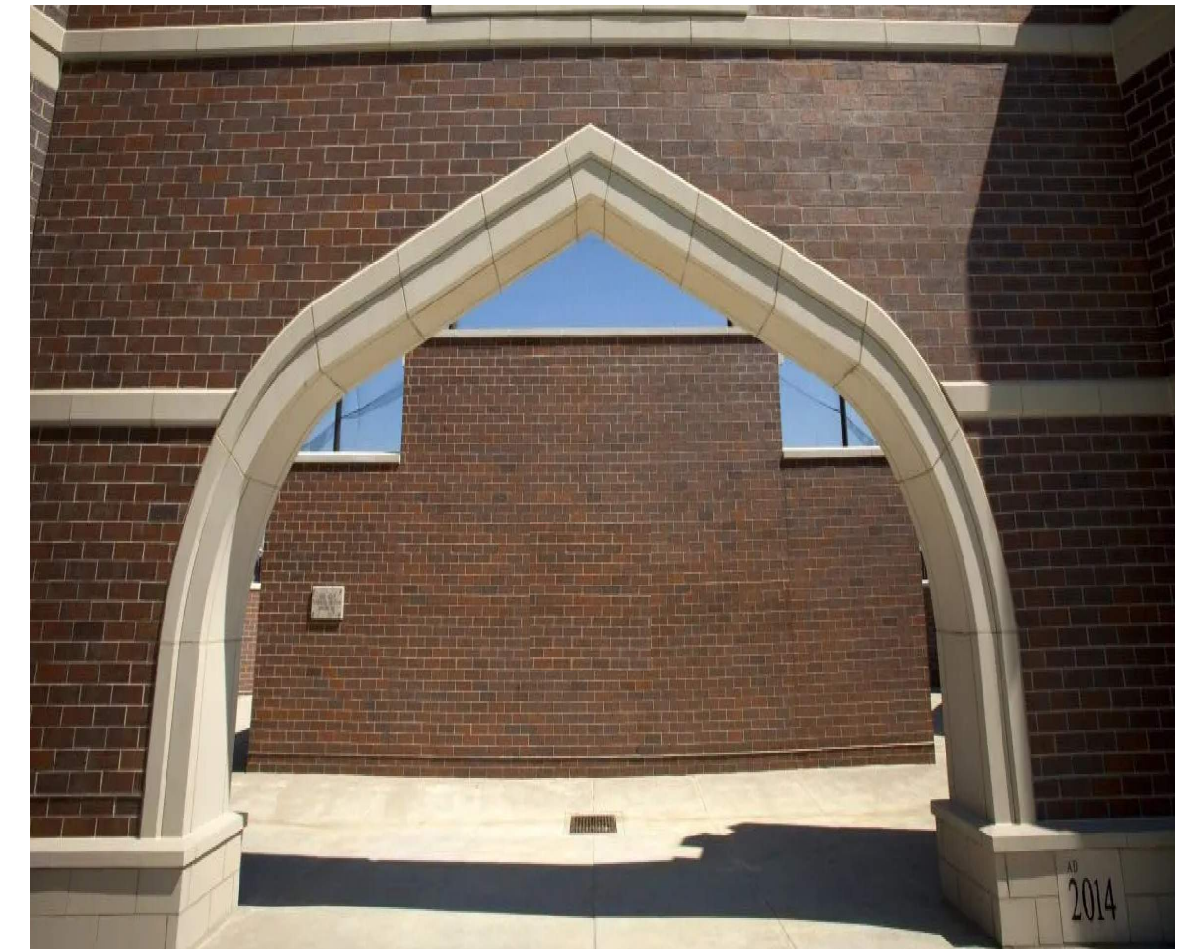
EXAMPLE: - BRICK - CAST STONE WATER TABLE - CAST STONE JAMBS, HEADERS & ARCHES - CAST STONE WALL CAPS.
