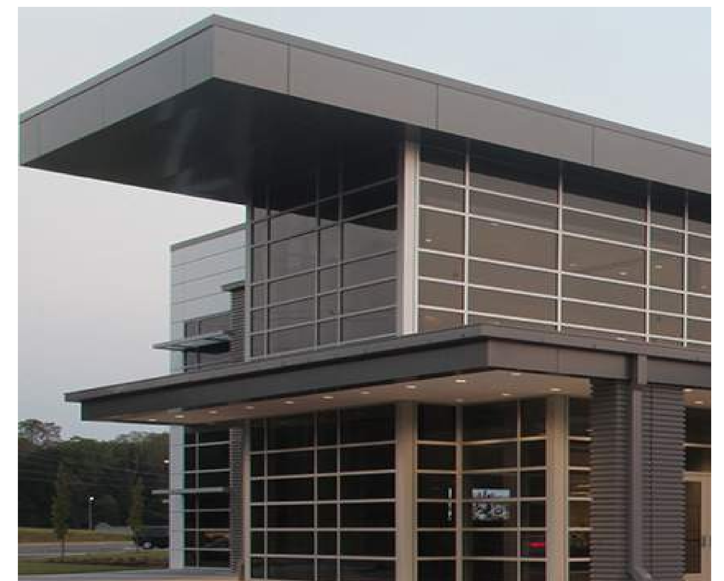
EXAMPLE: - PREFINISHED ALUMINUM COMPOSITE PANEL CANOPY SYSTEM - PREFINISHED ALUMINUM COMPOSITE PANEL ROOF SYSTEM - PREFINISHED ALUMINUM STOREFRONT FRAMING SYSTEM
