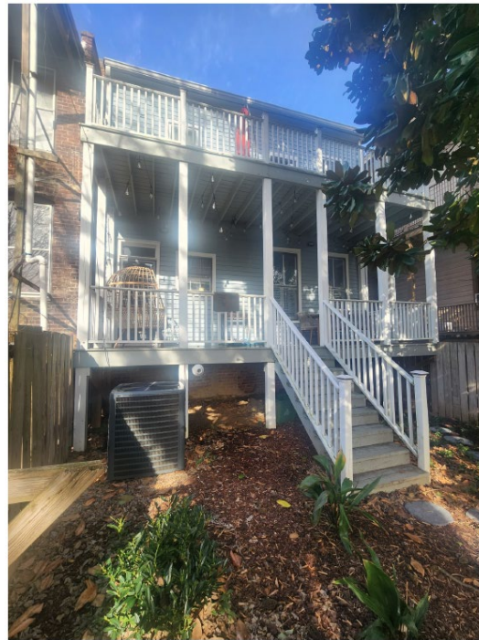
Figure 2: Existing back porch on 3009 E Broad St
