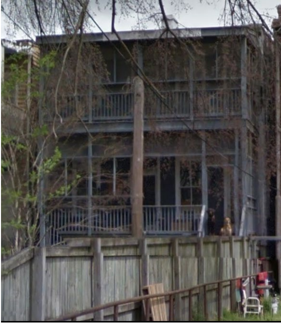
Figure 1: Back view of screened porch on 3005 E Broad St
