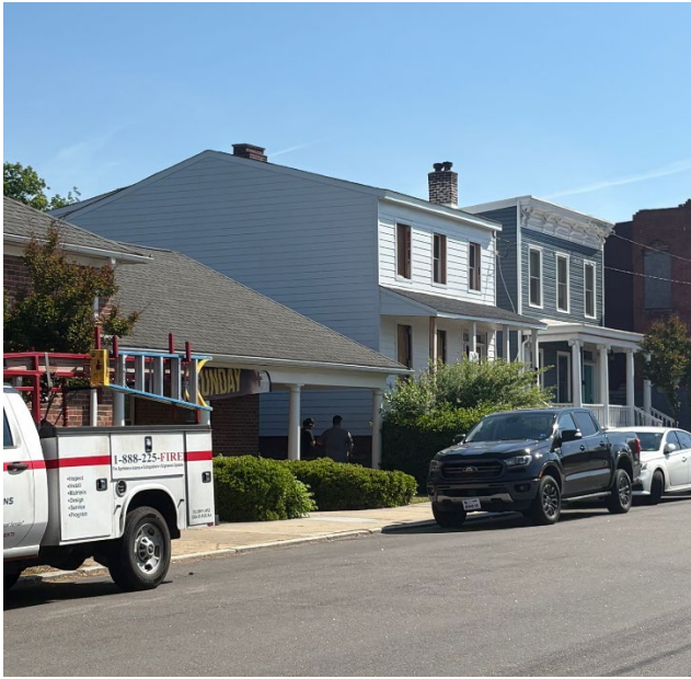
Figure 1. West elevation where windows will be installed. Existing conditions. April 2026.
