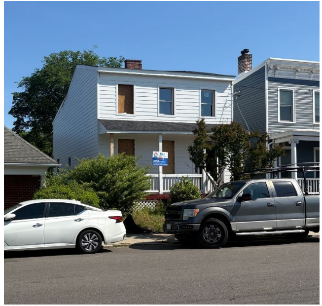
Figure 2. West elevation where windows will be installed. Existing conditions. April 2026.
