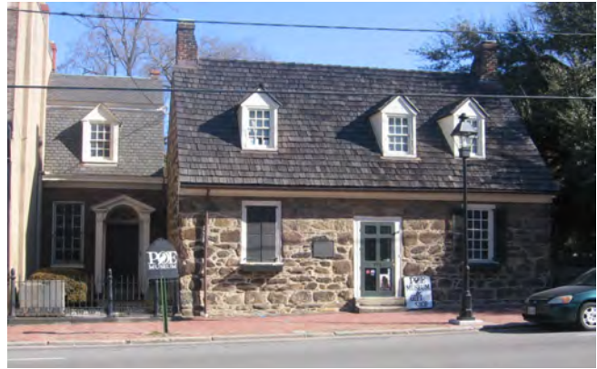
Old Stone or Samuel Ege House, built prior to 1783 1916 E. Main Street
