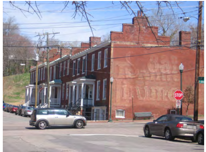
Elm Tree Row, built ca. 1853-1854 301-311 Cedar Street
