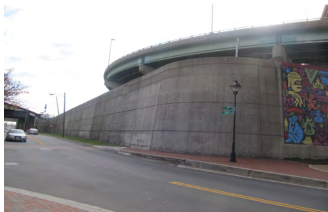
Richmond Floodwall, dedicated 1994
