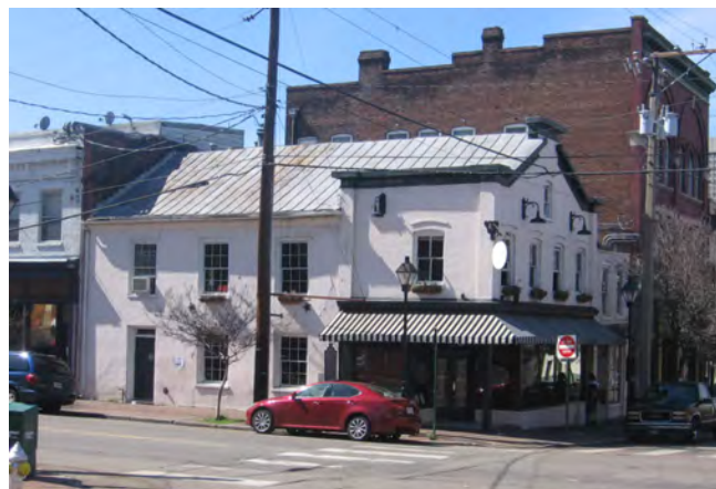
Whitlock’s Factory, built ca. 1817 1719 E. Franklin Street
