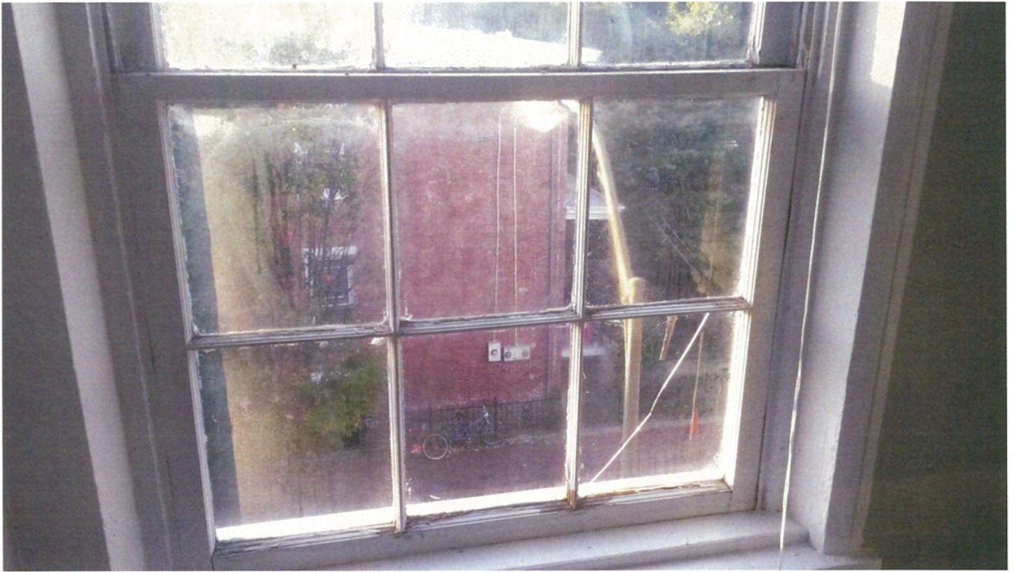
Glazing cracked.
