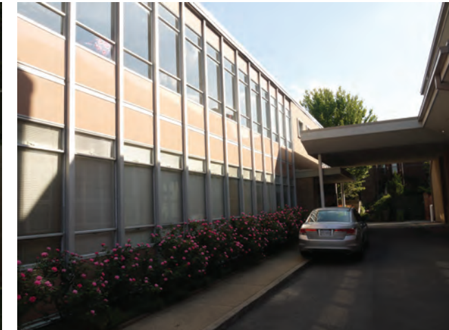
9| Side of 1121 and connection to 1125
