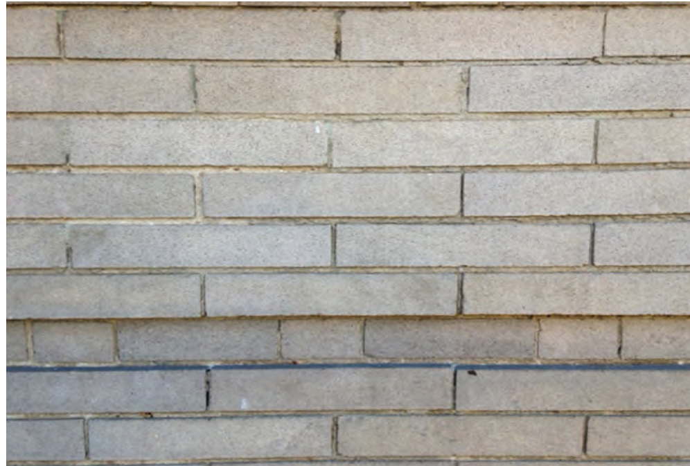
Existing brick at 1117 West Franklin St, Sanctuary Building
