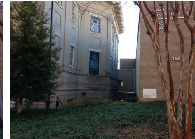
7| Close-up view of connection between 1117 and 1121
