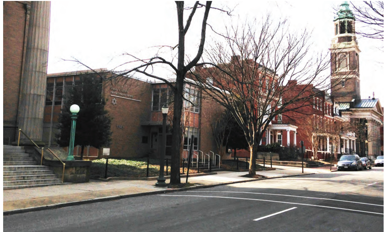
20| View of existing school facade from West Franklin St
