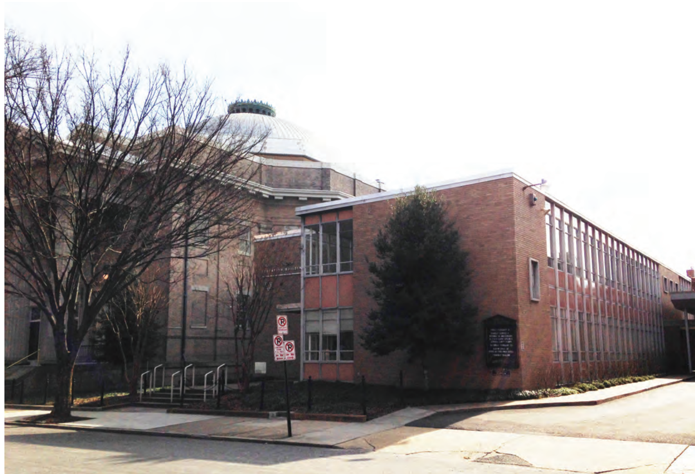
19| View of existing school facade from West Franklin St
