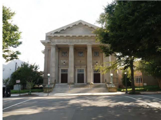
2| 1117 West Franklin St. - Sanctuary Building
