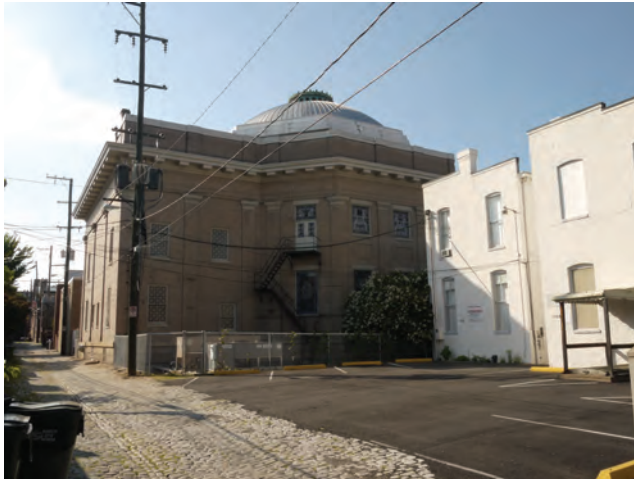
18| Alley view from 1109 and 1111, toward 1117 Sanctuary
