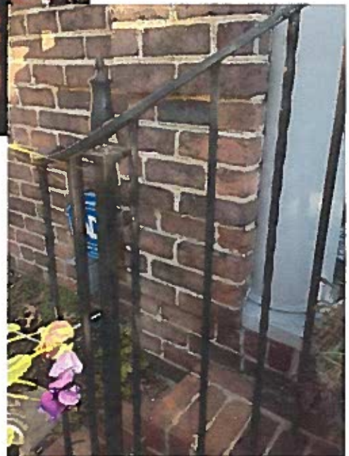
Front Railing Detail
