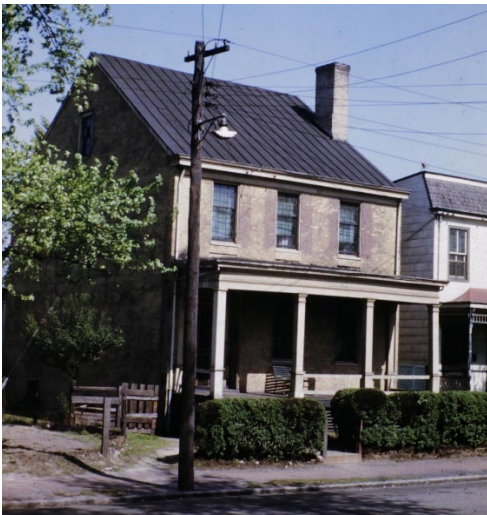
Figure 3. 510 North 29 th Street, circa 1941-1949. Valentine Archives, accessed January 16, 2024. Original Greek Revival style, covered front porch still present.
